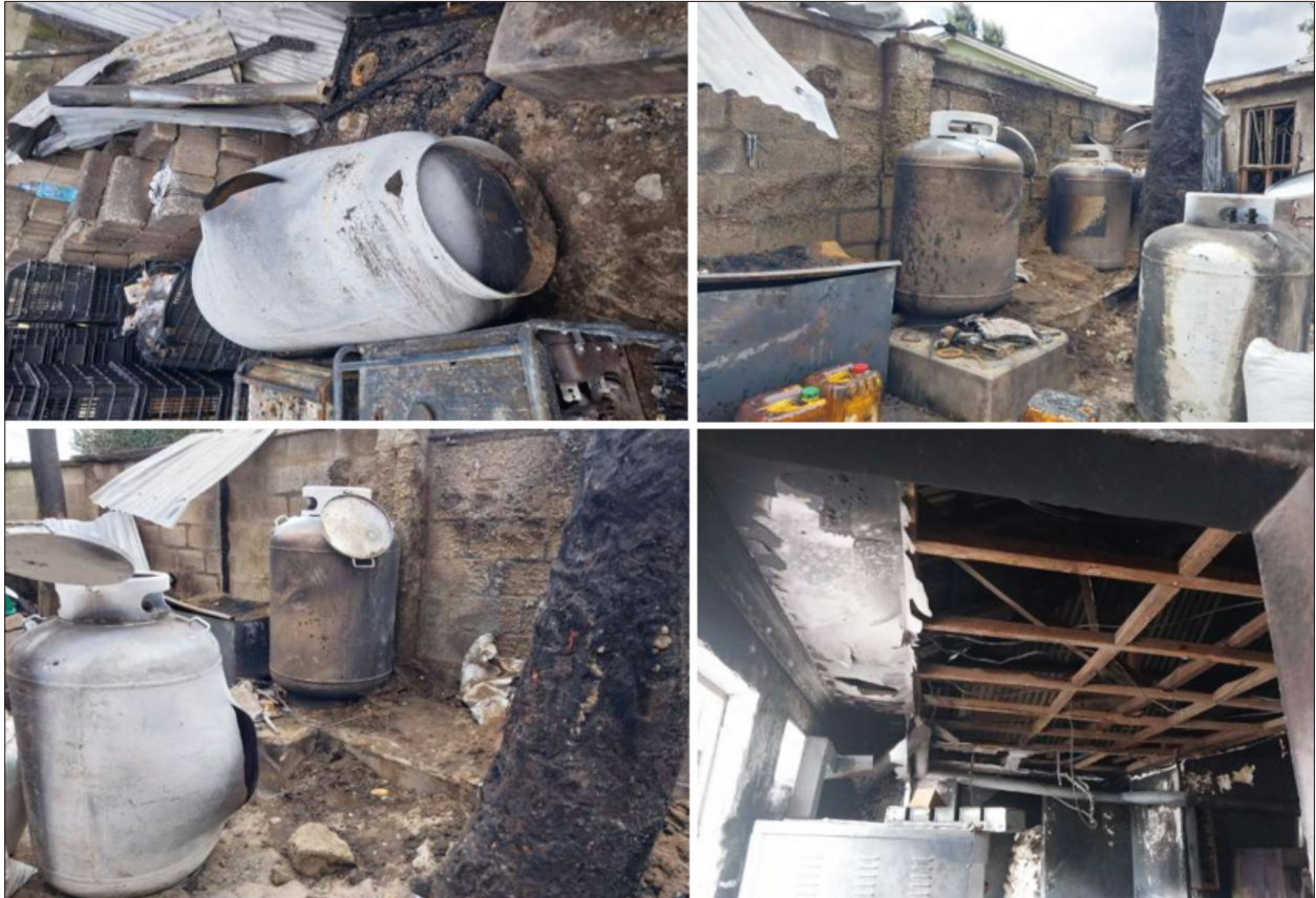
Figure 36: The LPG storage vessels incident at Keranyi village, Keranyi ward, Arumeru District in Arusha Region.
