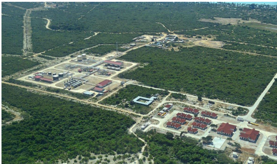
TPDC Songo Songo Processing Plant with a capacity of 140 mmscfd
